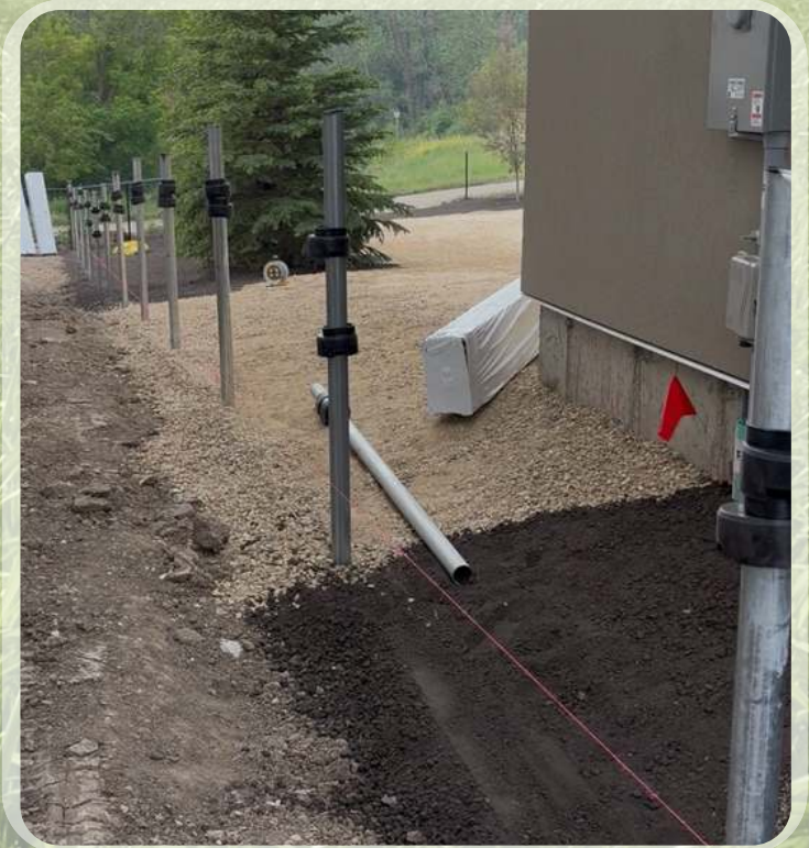
8ft Pipe Driven
